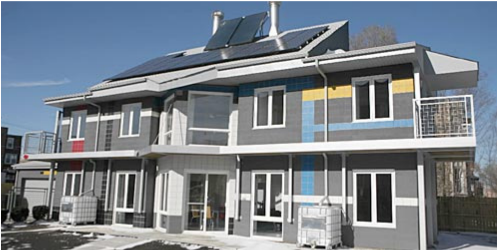
Architect Julian R. Dawson's home, in Chicago's Bronzeville neighborhood, includes large south-facing windows with insulated shutters that can be opened to admit passive solar energy. (Photo for the Tribune by Anthony Robert La Penna / January 30, 2008)
