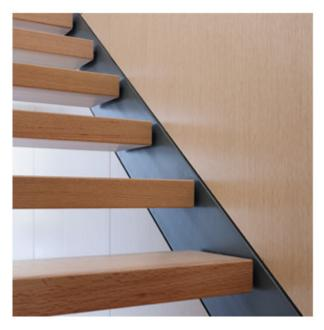
The staircase appears to float effortlessly from floor to floor. A steel channel stringer was recessed into the exterior gypsum-board wall on one side and the millwork on the other. Treads are composed of quartersawn red oak on ½-inch plywood that wraps around the steel plate running between the stringers, leaving a ¾-inch metal reveal on each end.
